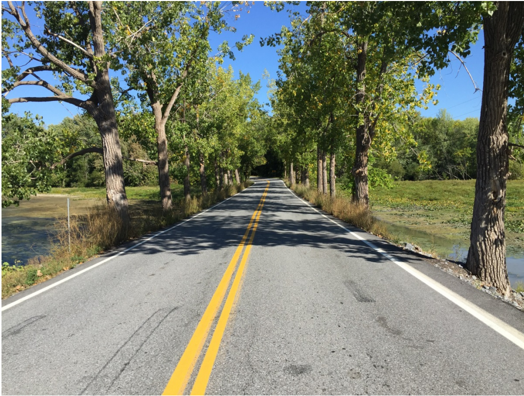
VT Route 125, Looking North
