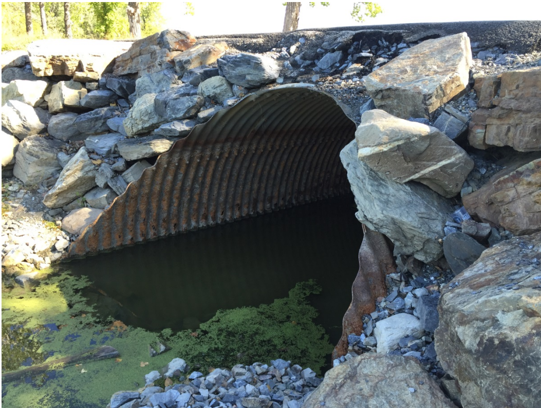
Culvert West Downstream End
