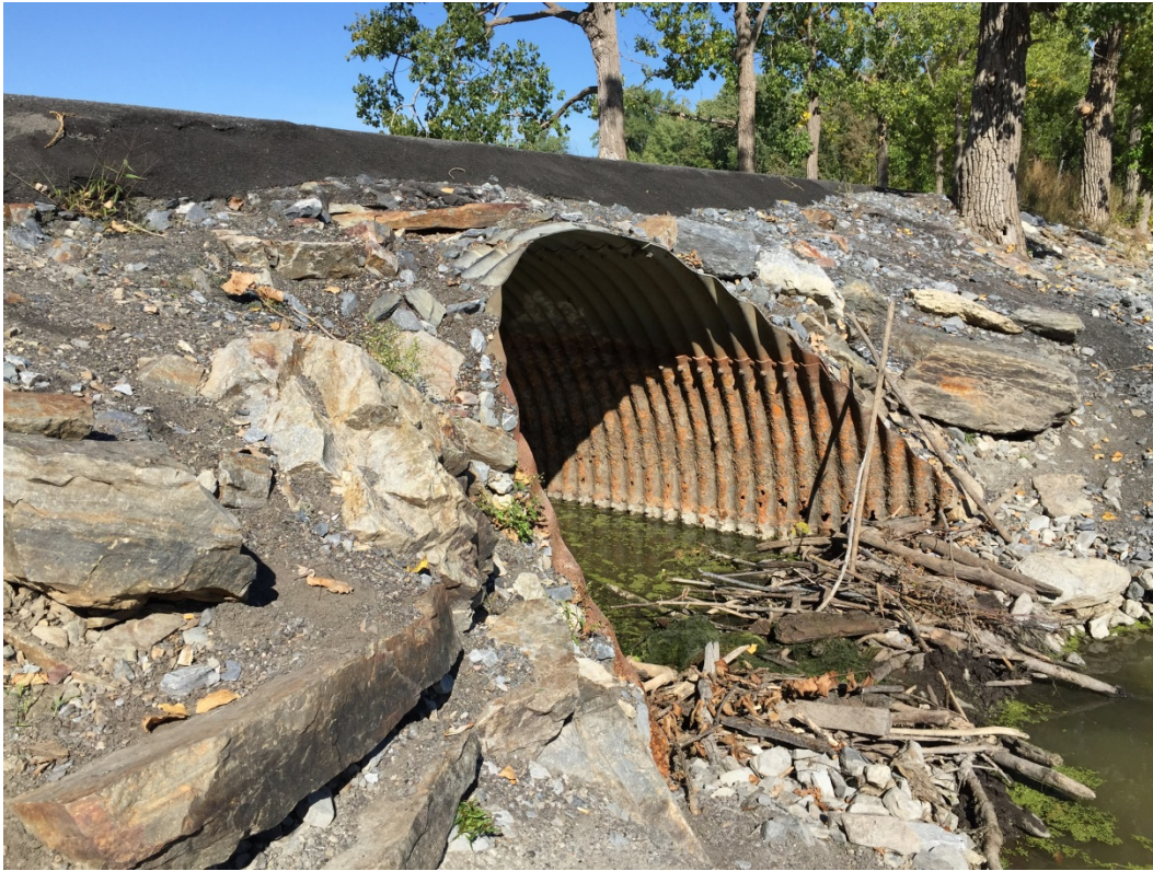
Culvert East Upstream End
