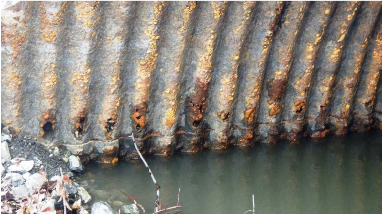
Figure 3: Inlet Corrosion
