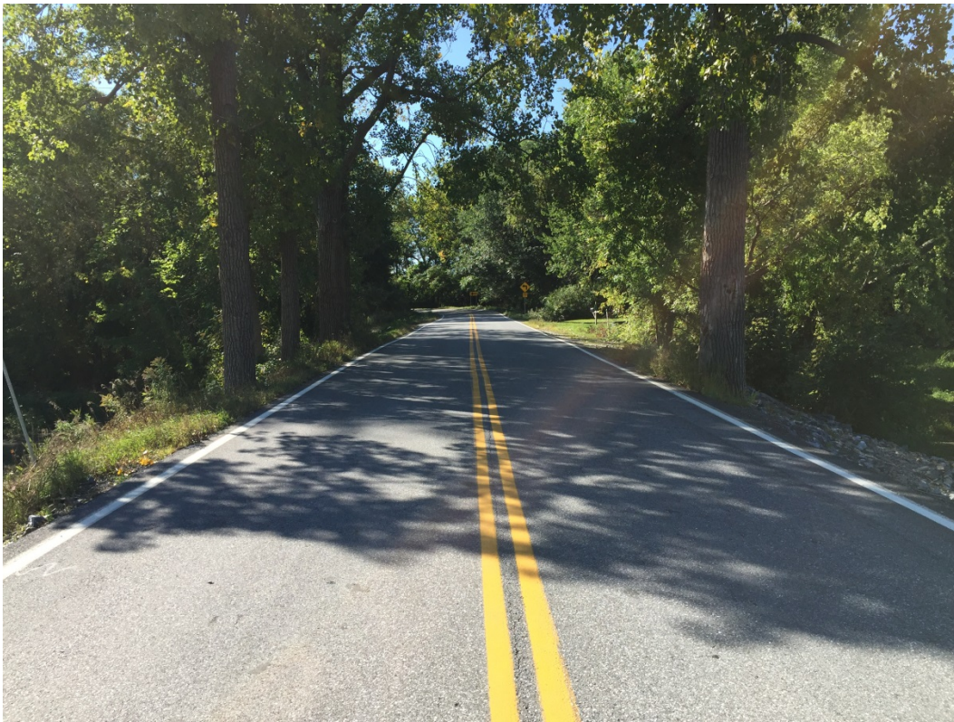
VT Route 125, Looking South
