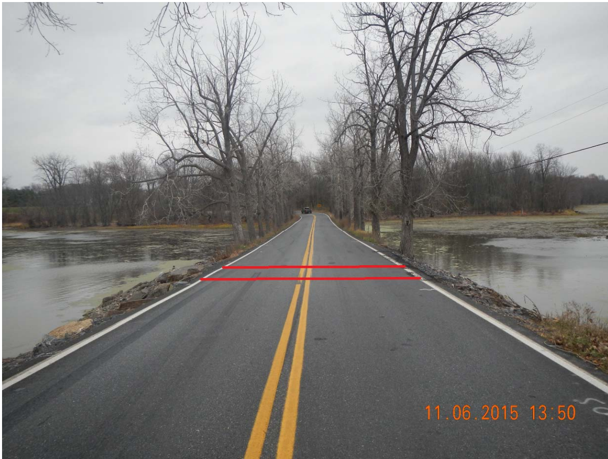
Figure 4: View at Culvert Location Looking North
