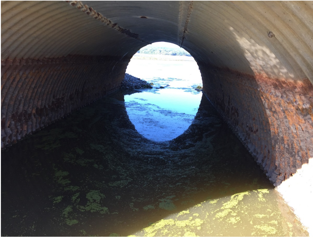
Looking West Downstream Through Culvert
